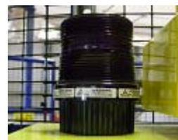
2. Over 20 mrad/hr: the magenta beacon will flash and the secondary shutter will close. An uncertified audible alarm was installed and may sound to draw attention.
