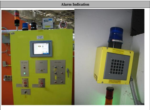
Stack Lights not illuminated Message display reads "02 Detector Fail Call PST 241-2727" and (depending on failure mode) blue strobes flashing Stack Lights not illuminated and (depending on failure mode) blue strobe flashing Audible alarm sounding
