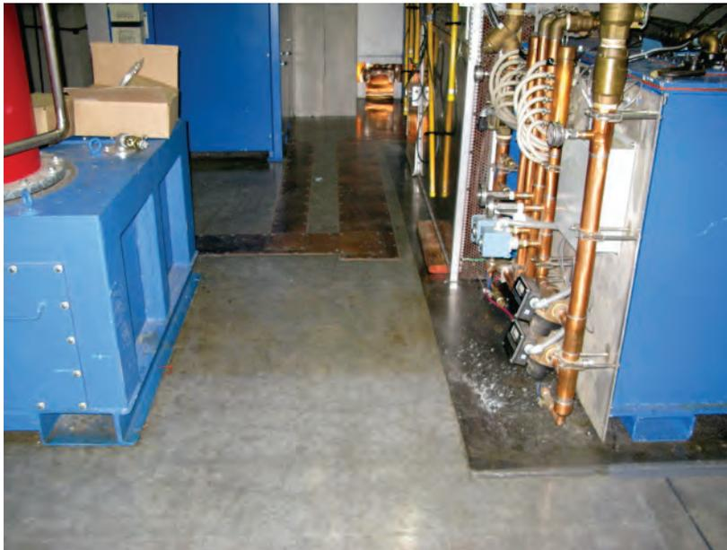
**Figure 4.41. Existing ground-plane installation in the Klystron Gallery.**
