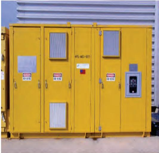
Outside 13.8 kV:2100 V 1.5 MVA transformer
